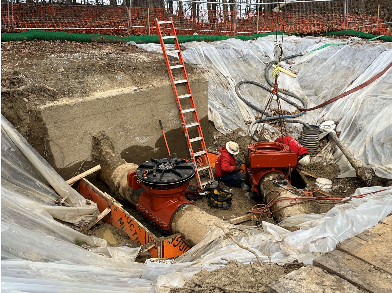
Installing New Valves on the Newington Side of the Little Bay Water Line
